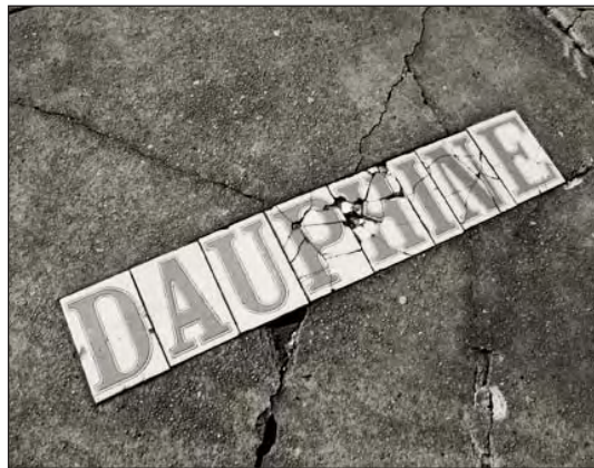
Ceramic tile marker at the corner of Dauphine and Piety. Such sidewalk-embedded street signs, dating from the late-nineteenth and early-twentieth centuries, are prevalent in New Orleans.
