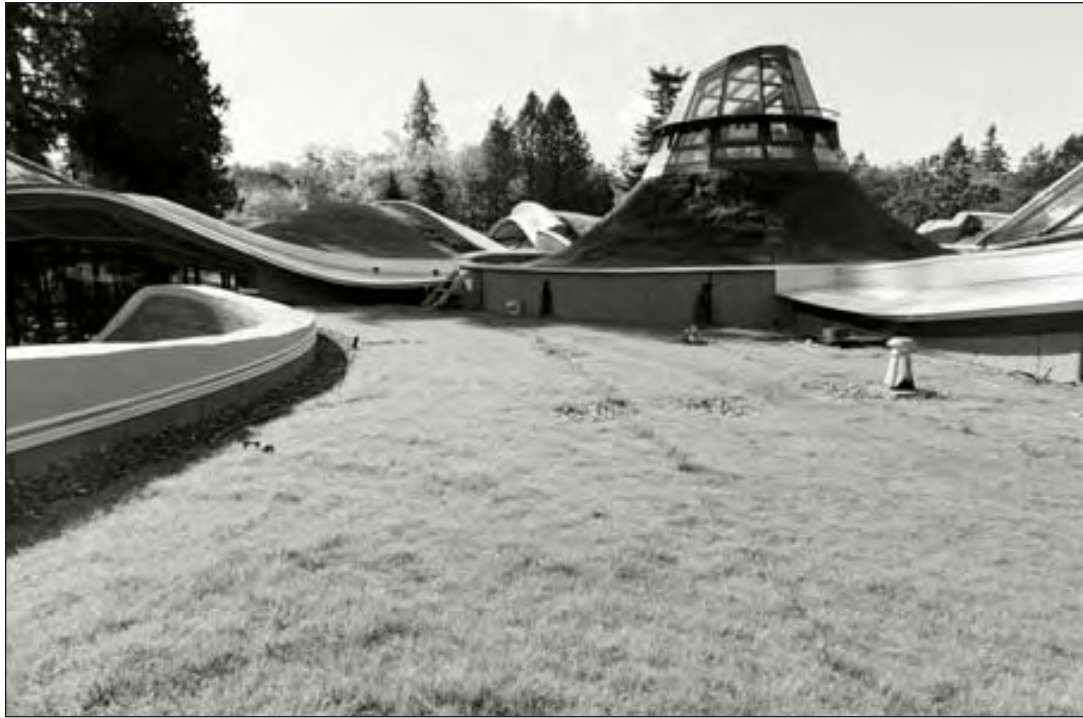
On top of the roof at the VanDusen Botanical Garden Visitor Centre (photograph by Stuart McCall/North Light).
