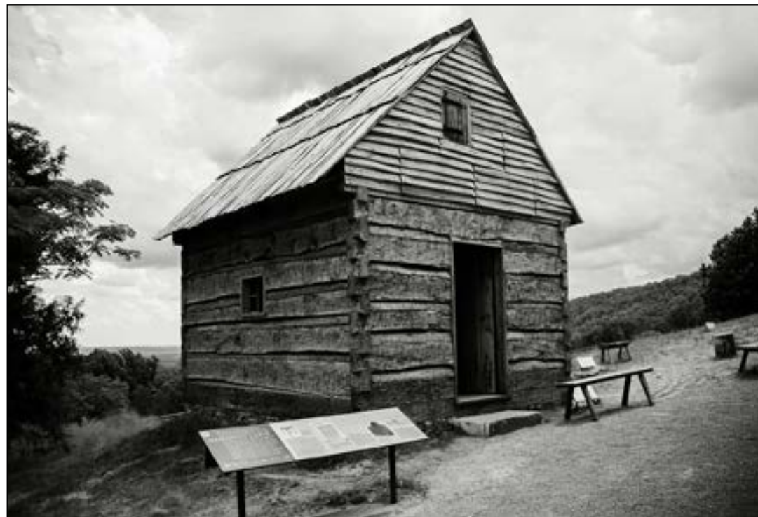
The reconstructed Hemmings Cabin.
